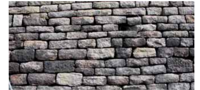
Wall at Stones, Todmorden
