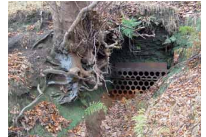
Coal mine entrance to adit, Gorpsey Clough
